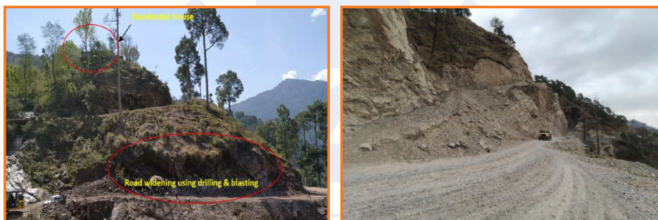
Fig. 1. View of some portions of Reasi-Arnas-Mahore (RAM) Road of BRO Road Projects, Jammu & Kashmir where safe widening of road using controlled blasting were implemented
