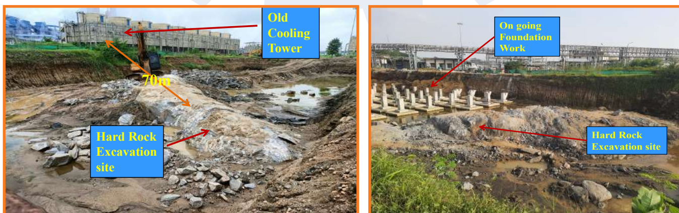
Fig. 3. Hard rock excavation site at a distance of 70 m from the old cooling tower
