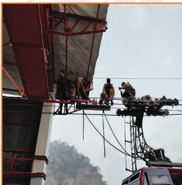
Non-Destructive Evaluation of Track Ropes and Haulage Ropes at Asia Resort Ltd. Timber Trail, Parwanoo, H.P.
