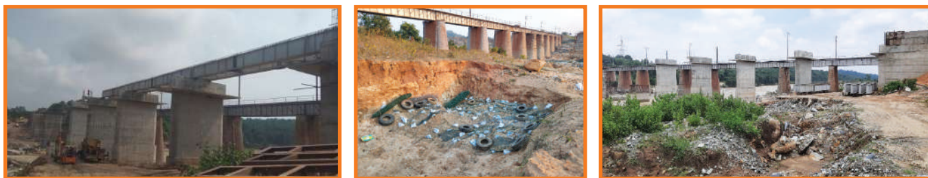
Fig. 4. View of controlled blasting works and piers installation for new railway bridge nearby the existing bridge at Koel river site of South Eastern Railway
